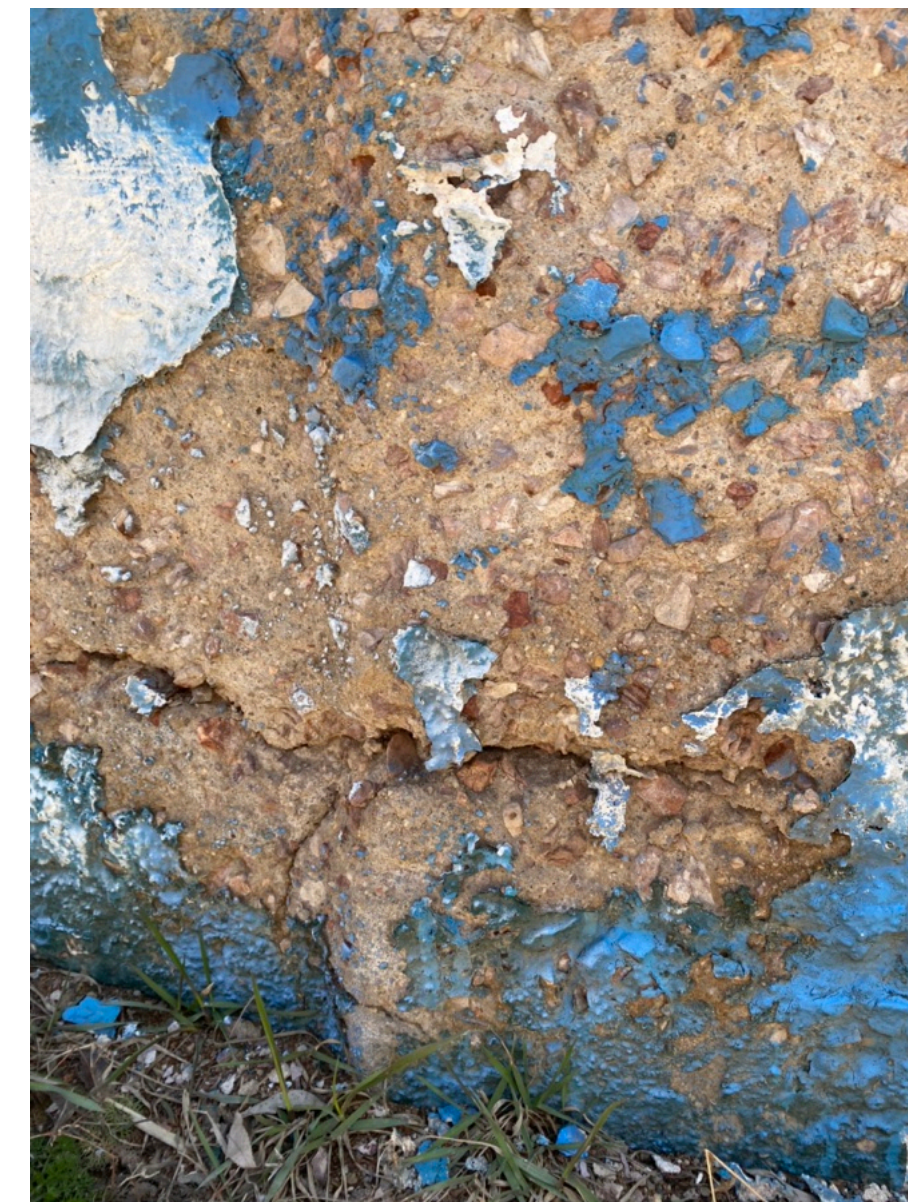
Top L & R, Bottom L - Examples of degraded concrete Bottom R - non street side of barricade
