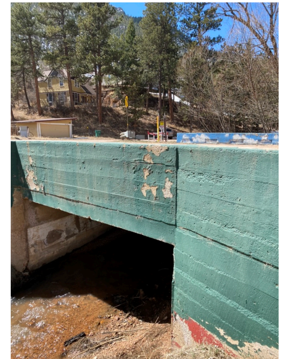
Top L & R, Bottom L - Examples of degraded concrete Bottom R - non street side of barricade
